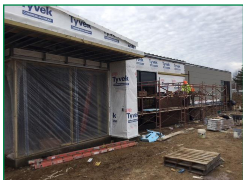
Brick exterior being installed on the Owensville branch.
