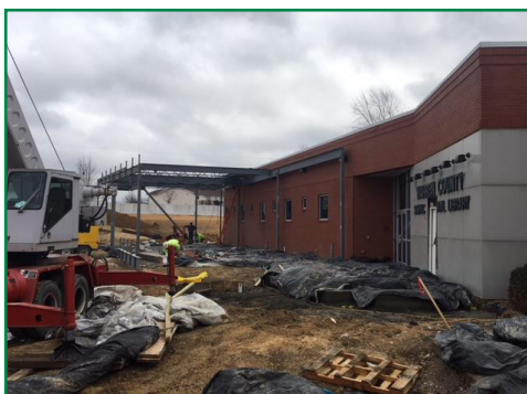
The steel frame being erected for the Warrenton branch expansion.
