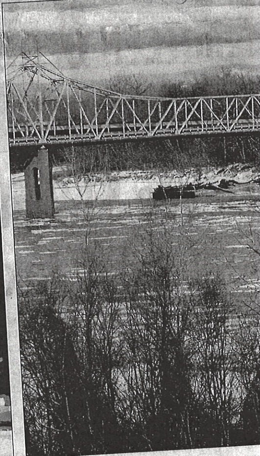
ICE FLOE UNDER BRIDGE Ice chunks floated in the Missouri River during a recent storm, moving west toward the old Highway 47 bridge. Crews are in preparation of imploding it in March. The d...
